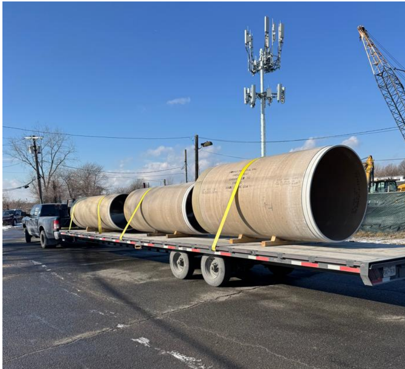
HOBAS Pipe Delivery 42-inch to 66-inch
