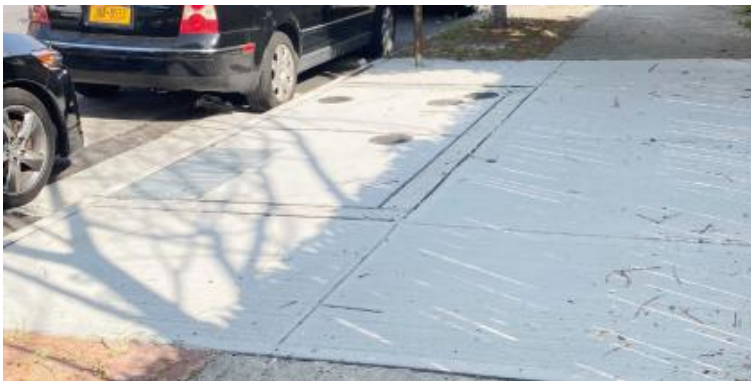
Infiltration Basin with Concrete Top
