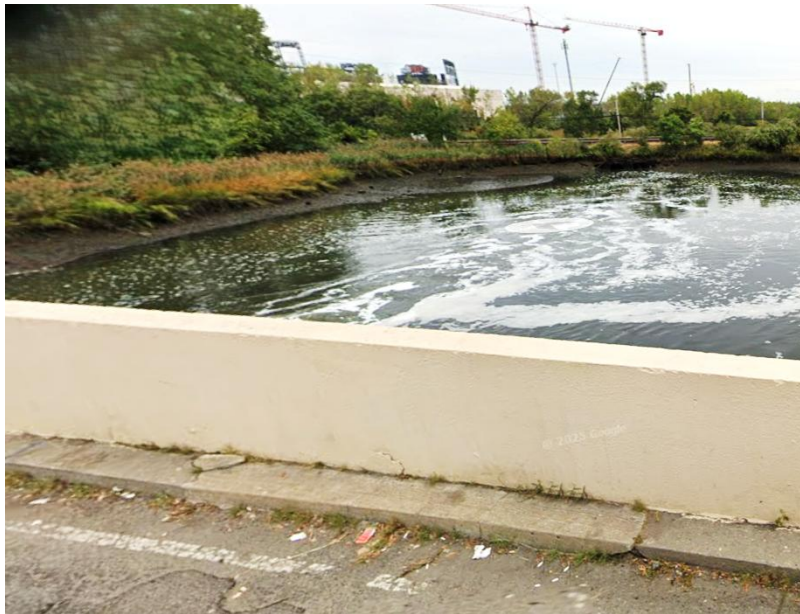
Parapet wall (south side of bridge) before demolition
