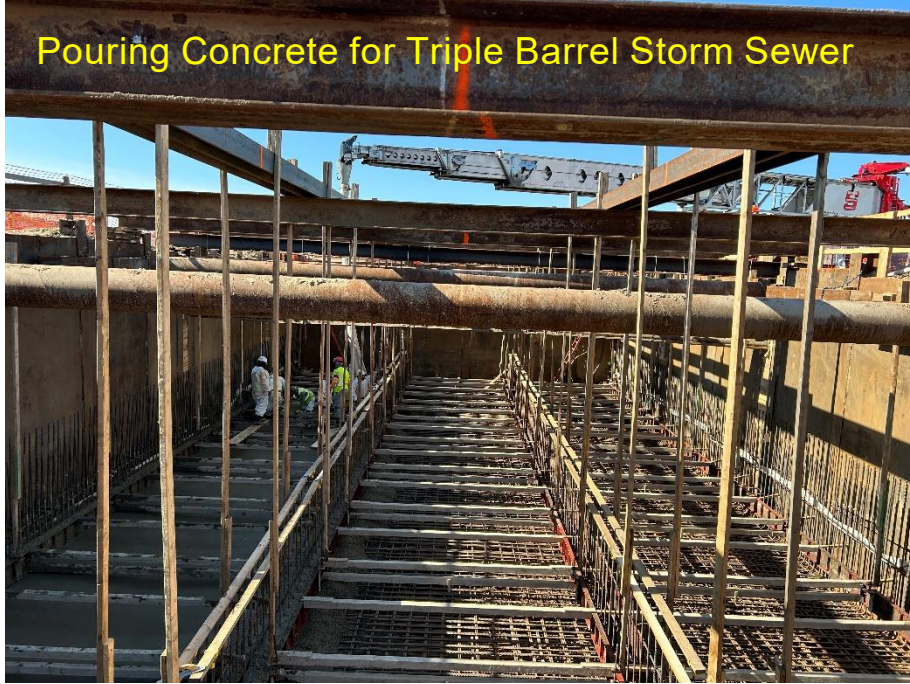
Pouring Concrete for Triple Barrel Storm Sewer
