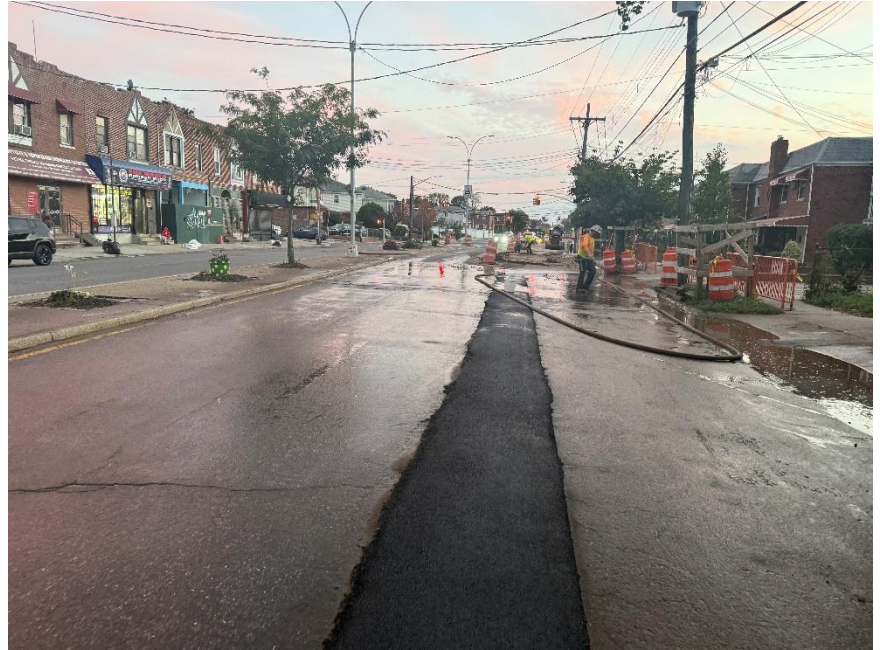
Springfield Boulevard water main installation
