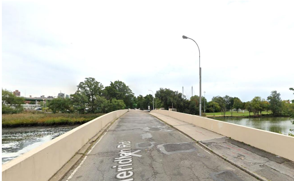
Bridge deck (east side of bridge) before demolition
