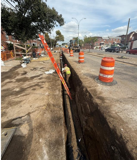
Springfield Boulevard water main installation
