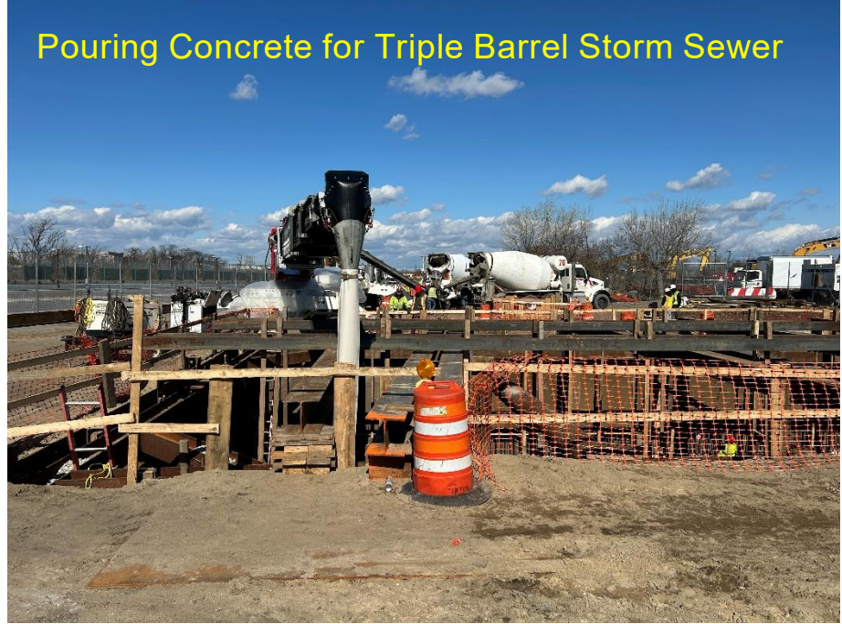
Pouring Concrete for Triple Barrel Storm Sewer
