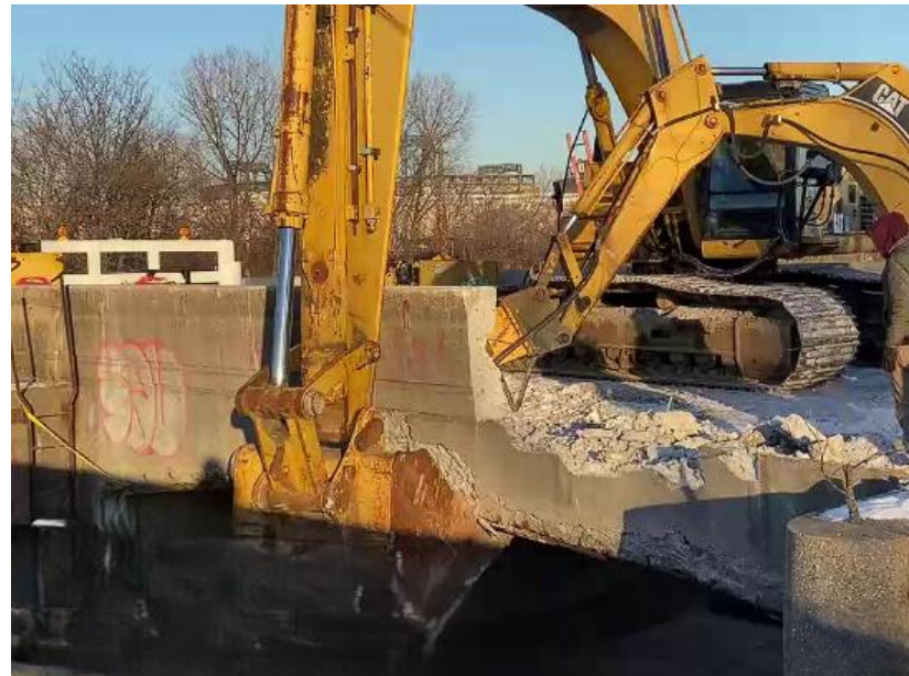
Parapet wall (south side of bridge) demolition
