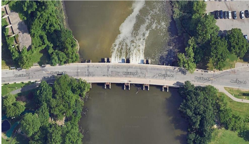
Bird's eye view of the Tide Gate Bridge prior to demolition
