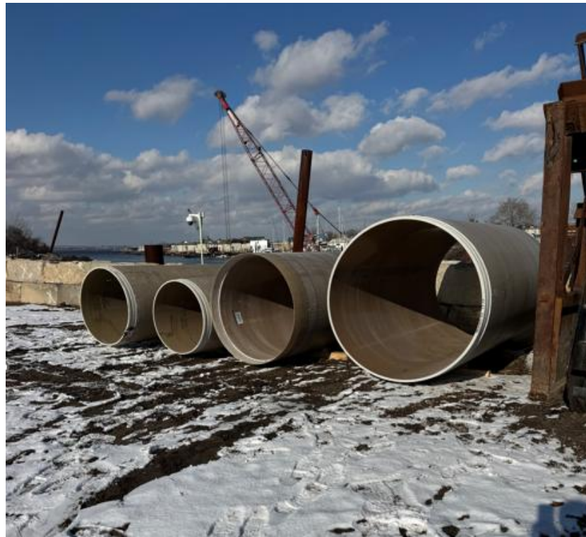
HOBAS Pipe Delivery 42-inch to 66-inch
